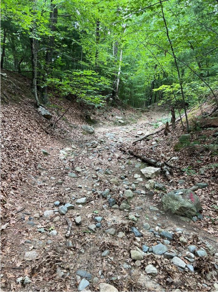
7 Section of the Warner Trail displaying need for soil stabilization.
