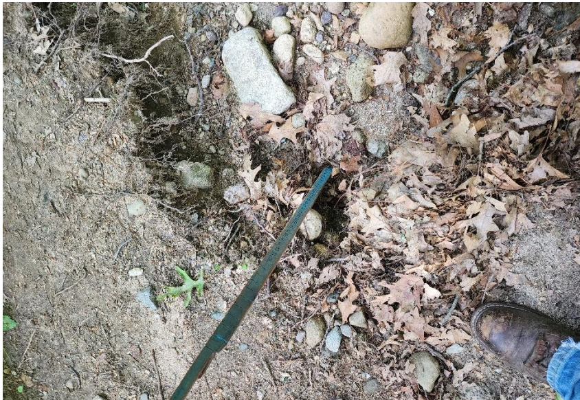
6 Washed out section of the blue trail due to surface flow.
