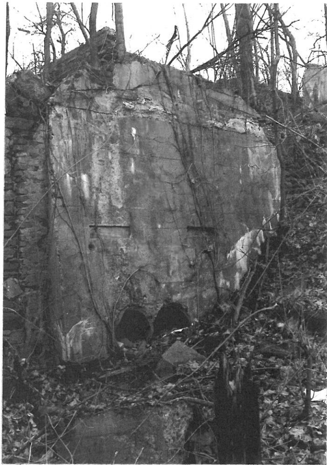
Plate 2. CONCRETE IN-FILL AT PROBABLE HEADRACE ARCH SITE, HARRIS MILL Concrete section about twelve feet wide; surviving springline voussoir at extreme left center. View is to northeast.
