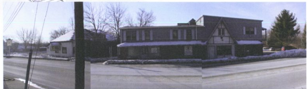
EXISTING SITE CONDITIONS
