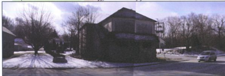
EXISTING SITE CONDITIONS
