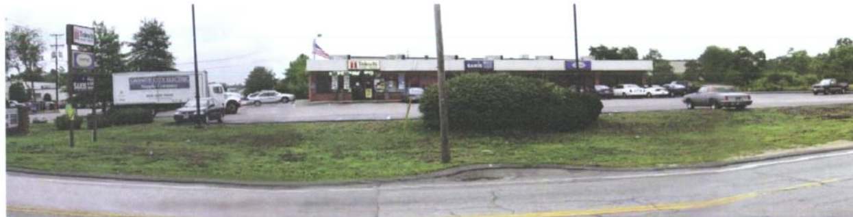
EXISTING SITE CONDITIONS
