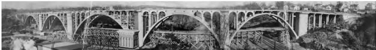
Ashton Viaduct Bridge ca. 1935
