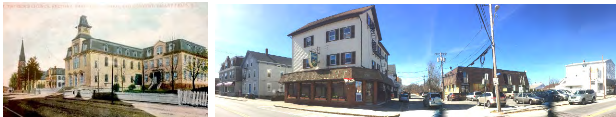
St. Patrick's Church (ca. 1890) and Broad Street today, notable for vinyl clad period buildings, infill and vacant lots.
