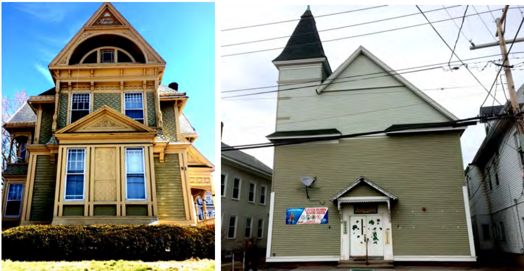
Contrast on Broad Street: restored John F. Clark House (1882) Queen Anne versus vinyl cladding, which obscures historic architectural details
