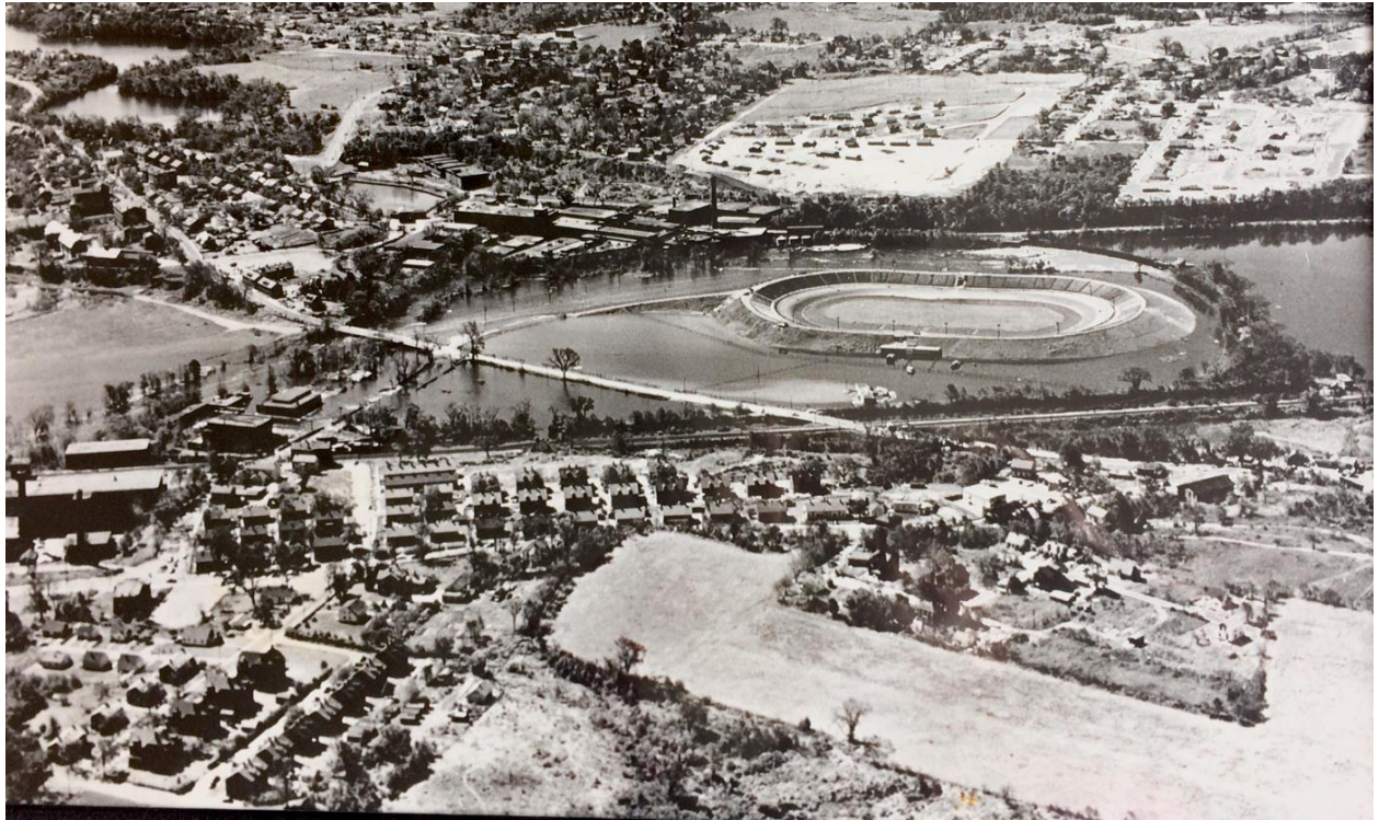
Lonsdale, ca. 1954, during a flooding event (likely Hurricane Carol). The northern area, to the right of the Lonsdale Sports Arena, is now the OU2 Nunes parcel.
