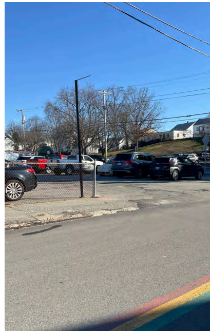
High Street bituminous sidewalk showing failure and no ADA ramp
