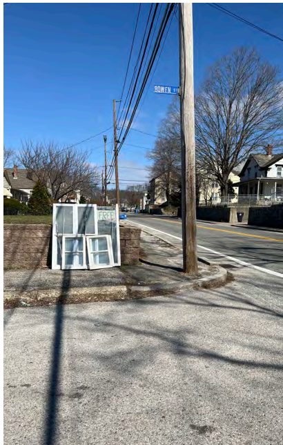
Lack of ADA ramp (High Street/Bowen Street intersection)
