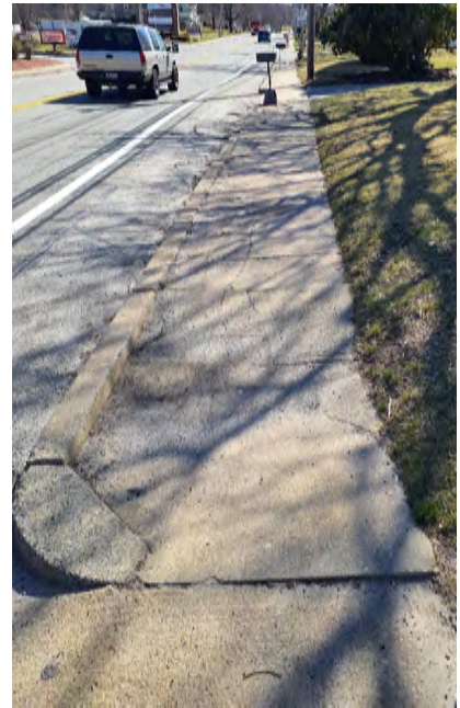
Settled section of concrete sidewalk creating tripping hazard (Mendon Road)
