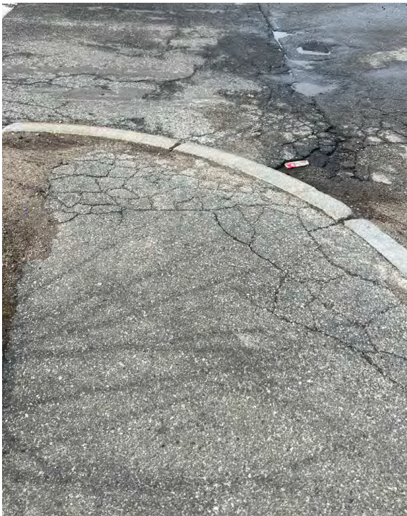
Cracked asphalt and lack of ADA ramps on Dexter Street
