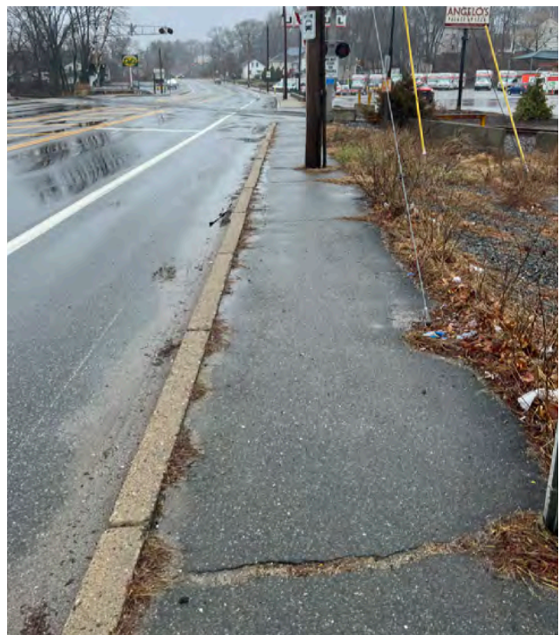
Area of sidewalk on Mendon Road by Stop & Shop with significant cracks and ADA issue due to clearance.
