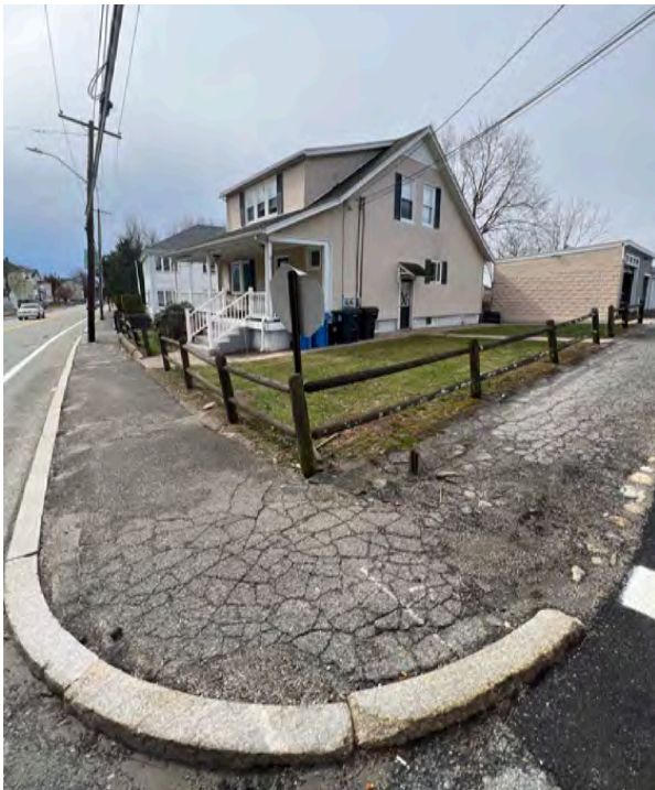
Section of High Street with sidewalk in poor condition with extensive cracking and no ADA ramp
