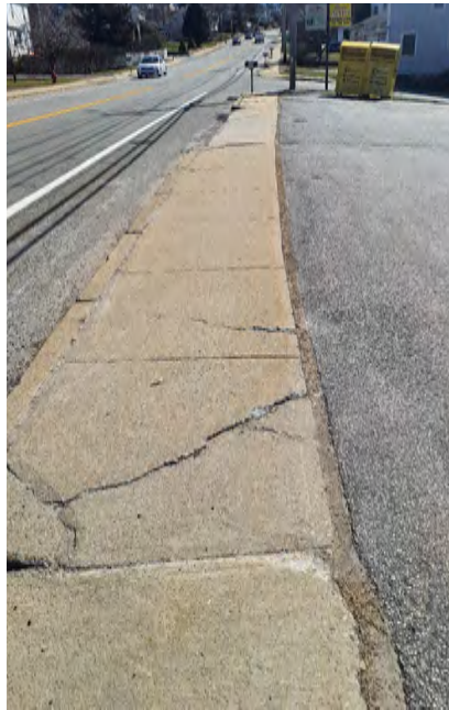
Section of cracked concrete sidewalk (Mendon Road)
