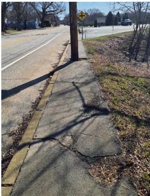
Failed sidewalk and ADA issues on Pine Swamp Road
