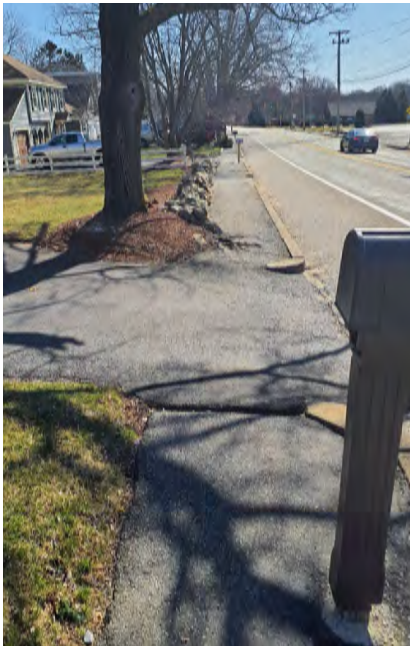
Tree roots impacting safe passage (Pine Swamp Road)
