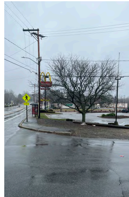
Lack of ADA ramp (Mendon Road by Stop & Shop)
