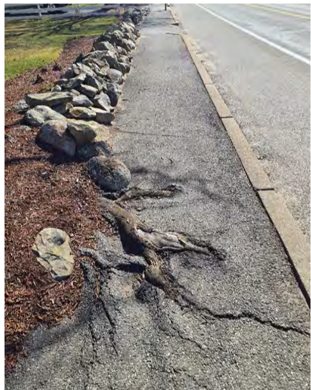
Tree roots impacting safe passage on sidewalk on Pine Swamp Road
