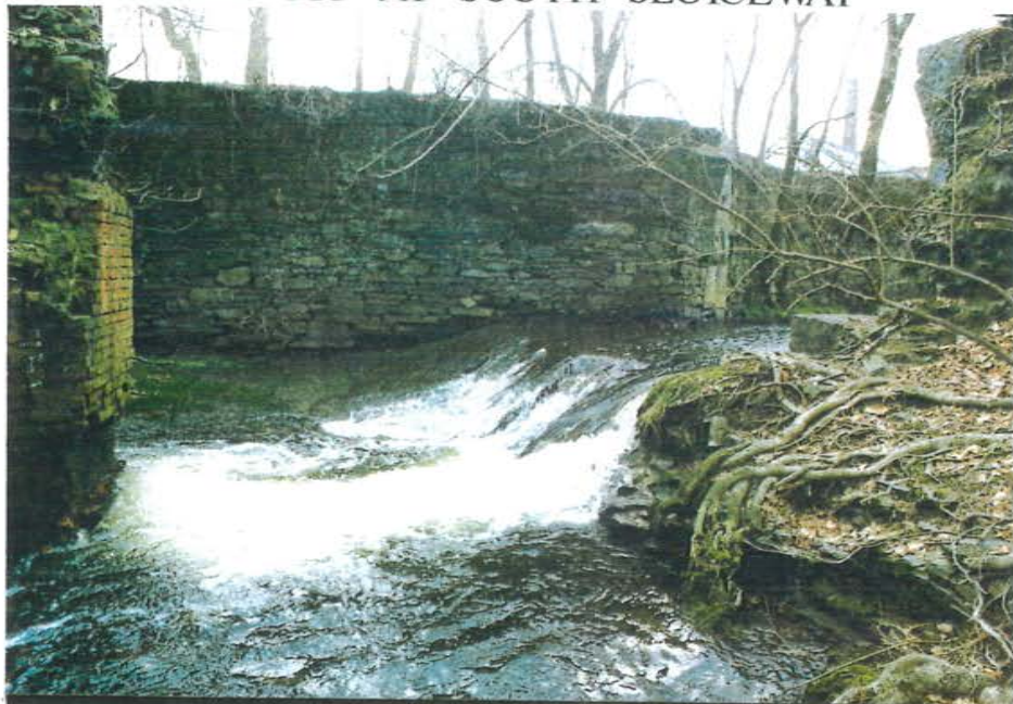
J - TURBINE PIT AT SOUTH SLUICeway
