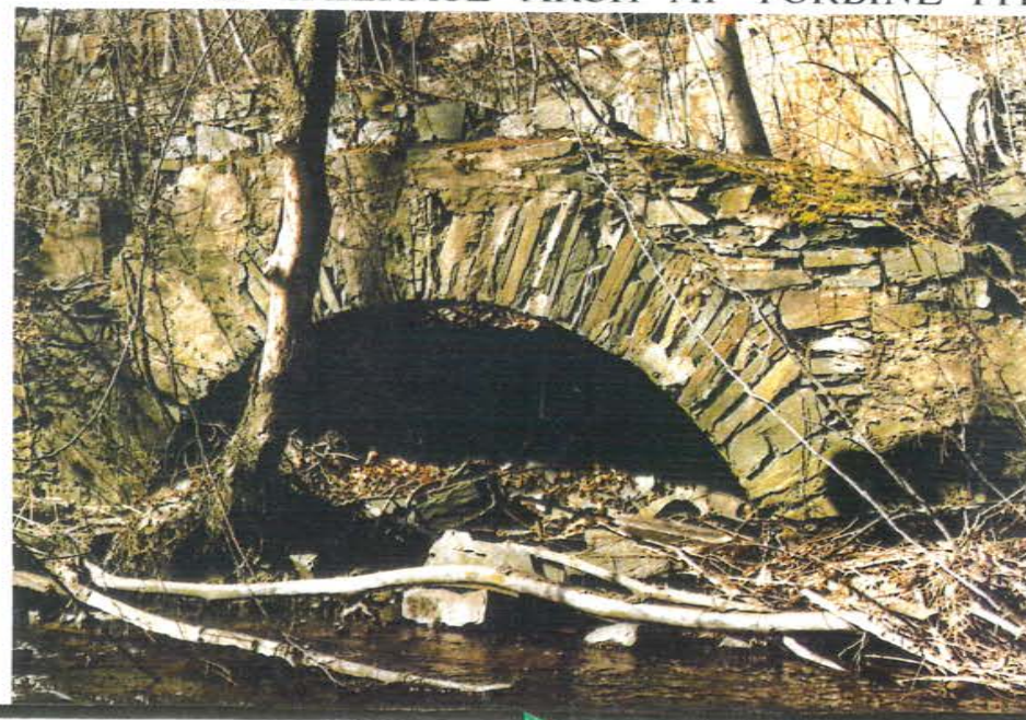
L - TAILRACE ARCH AT TURBINE PIT
